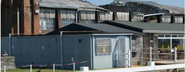
From the south - single story buildings are generally post 1980. The former Flight Commanders office is to the right - see subsection B for fuller description of this building.
