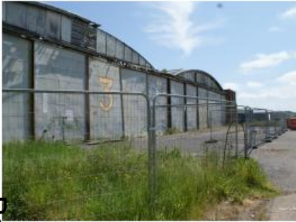
May 2023 Hangar 3 southern elevation
