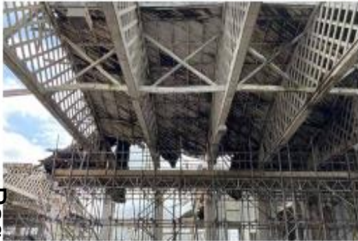
Belfast trusses remaining in-situ
