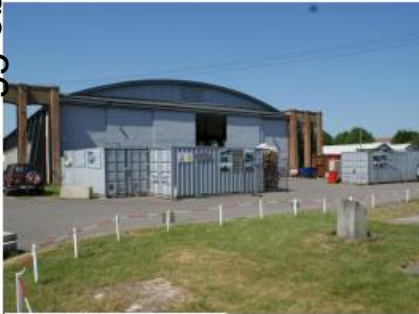
May 2023 Hangar 4 near elevations from aerial
